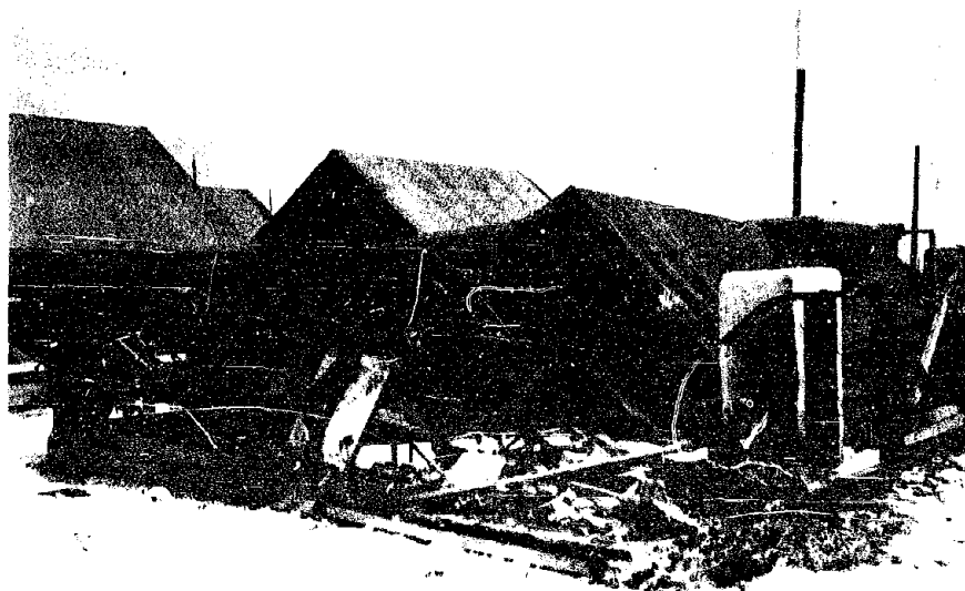
Fig. 3.7. Typical Damage to Four-man Tents, Tare Island, Postshot, 14-3/4 Miles from GZ
